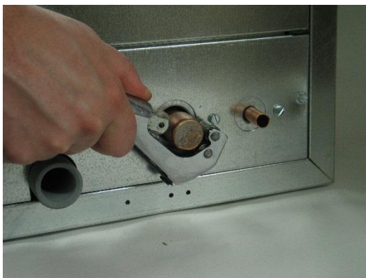
Figure 21. Cut end of connection as shown.
