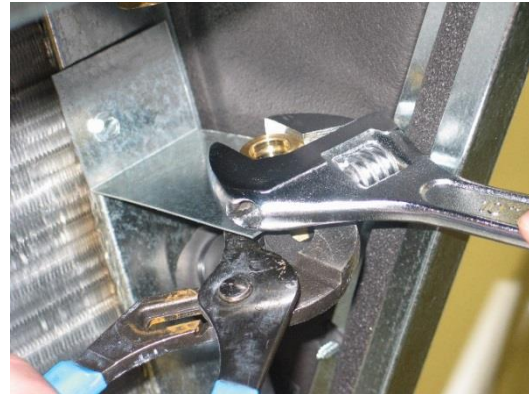
Figure 22. Remove Nut
