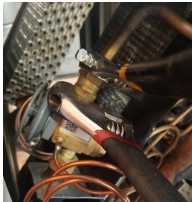
Figure 24. Attach and tighten upper connecting nut (B/E coils)
