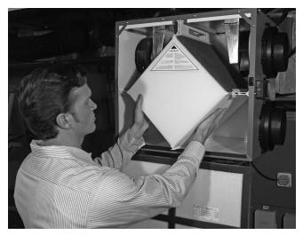
2. Open the side door panel by opening the two latches on the top of the side panel and lowering the panel to its fully open position Remove both filters from the top left and right sides of the Core, then vacuum both filters.
