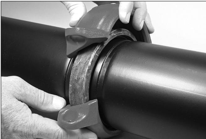
**5. INSTALL HOUSINGS:** Install the housings over the gasket. Verify that the housings’ keys engage the grooves completely on both mating components.
