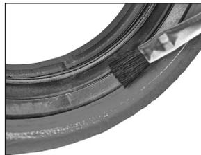
**3a. IF ANY CONDITIONS LISTED IN THE NOTICE BELOW ARE MET, APPLY A THIN COAT OF A COMPATIBLE LUBRICANT ONLY TO THE GASKET SEALING LIPS:** For EPDM gaskets, use Victaulic Lubricant or an EPDM-compatible lubricant. Silicone grease may be used (silicone spray is not a compatible lubricant).
