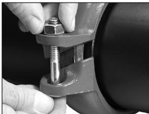
**6. INSTALL REMAINING BOLT/ NUT:** Install the remaining bolt, and thread the nut finger-tight onto the bolt. **NOTE:** Verify that the oval neck of each bolt seats properly in the bolt hole.
