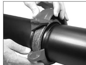
5. **INSTALL HOUSINGS:** Install the housings over the gasket. Verify that the housings’ keys engage the grooves completely on both mating components.
