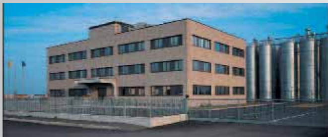
Production, Operations & Administration Centre- Castel Guelfo di Bologna (BO) Italy
