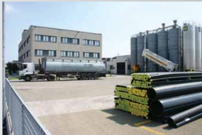
Production, Operations & Administration Centre - Castel Guelfo di Bologna (BO) Italy
