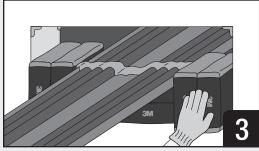
Install  $3M^{\text{\tiny{M}}}$  Fire Barrier Pillows or Self-Locking Pillows, starting along one side of the opening using the largest size possible. Pillows should be tightly butted, with a minimum of 25% compression from their original thickness, and installed with the 3M logo facing out such that the longest length projects through the opening. Pillow should be centered through the opening where applicable.
