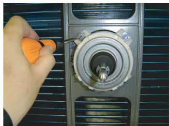
Remove the 4 mounting screws.
