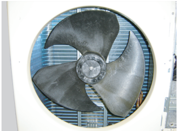
Remove the nut. And remove the PROPELLER FAN. Note at the installation. Insert propeller Fan and Moter shaft reference D cutting position. And the tightening torque at the installation. Tightening torque is from 10 to 12N-m.
