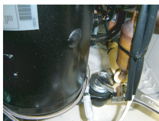
Remove the COMP BOLTS. (3 places)
