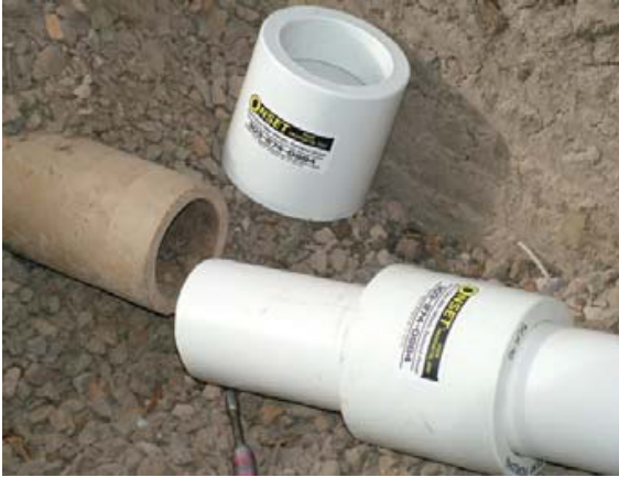
Step 1 Slide the Shear Guard™ support onto exposed pipe that is to be joined to existing pipe.
