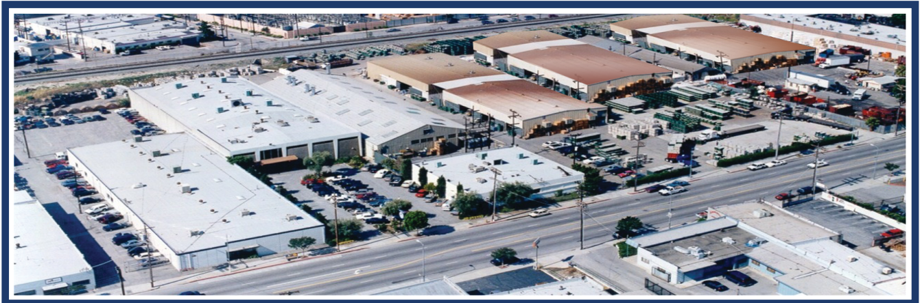
Corporate Facility / North Hollywood, California
