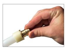
4. Insert fitting into expanded tube and sleeve. Hold fitting in place until tube/sleeve constricts annularly around the fitting.
