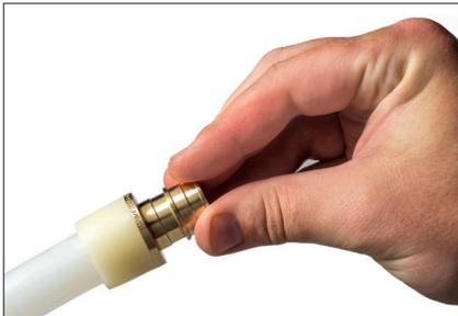
4. Insert fitting into expanded tube and sleeve. Hold fitting in place until tube/sleeve constricts annularly around the fitting.
