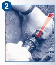
Insert the pipe until the first point of resistance is felt.
