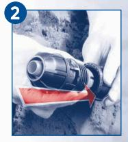
Assemble the fitting by pushing the fitting body over the insert and sliding the collet and the nut up to the insert shoulder.
