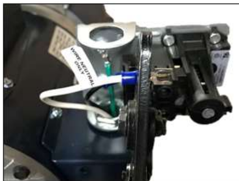
5. Crimp a spade connector onto NEUTRAL wire.
