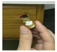
Once the wires are firmly connected, you can firmly press the round button into the hole until secure.
