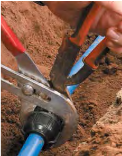
4. Nut Tightening
