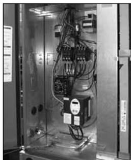
For added convenience in the field, a factory-installed convenience outlet (13) is available. Low and High voltage can enter either from the side or through the base. Low-voltage connections are made integrated cooling control. The high-voltage connection is terminated at the number 1 compressor contactor. The suggested mounting for the field-installed disconnect is on the exterior side of the electrical control box.
