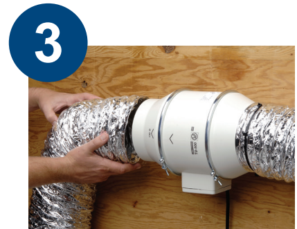
Connect the ducts.
