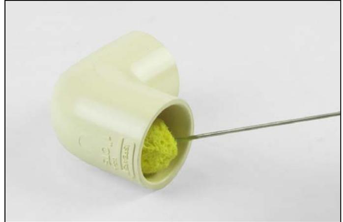
Apply a medium coat to the fitting socket. Avoid getting cement in other sockets or threaded connections. A second application of cement must be applied to the pipe end if a 1-1/4 inch and larger joint is being prepared.
