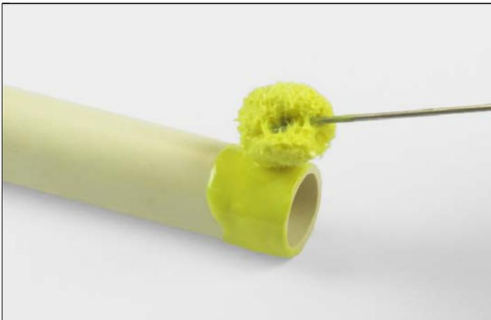
Apply a heavy, even coat of cement to the outside of the pipe end. Work the cement into the joining surfaces using a continuous, circular motion.
