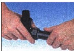
2. Push the fitting onto the pipe up to the housing of the white circlip.
