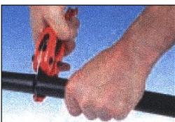
1. Square-cut the poly pipe to the required length with pipe cutters, knife, or saw.
