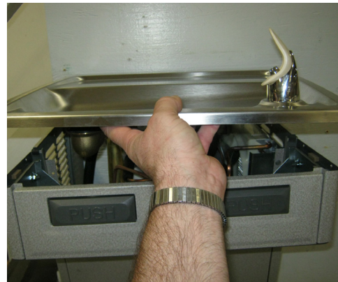
Lift and Remove Basin.
