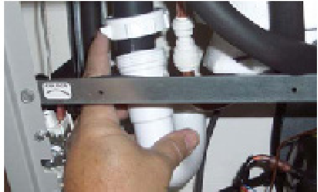
Reattach drain line to P-trap
