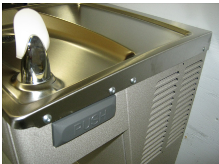
Remove Basin Fasteners
