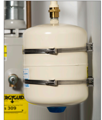
Double Band Wall Installation
