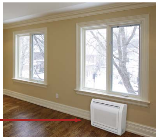
At less than 24" high and 30" wide, floor mount models fit easily under a standard window and can replace a radiator twice its size while producing more capacity.
