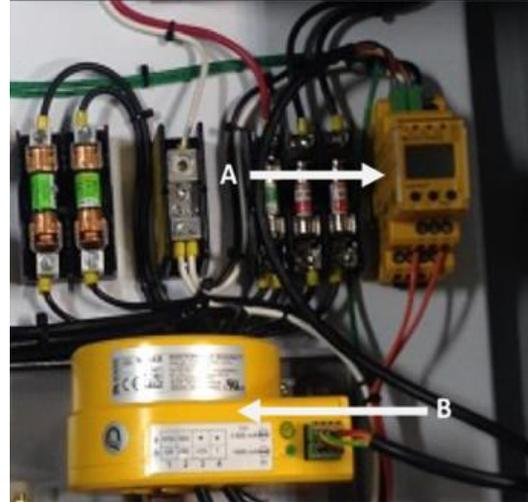
Test and reset functions are carried out automatically every 24 hours. To manual test the GFCI, press the test button for a minimum of 1.5 seconds. To reset a tripped GFCI, cycle the power of the unit. If equipped with a disconnect handle, turn the handle to the "OFF" position then back to "ON".
