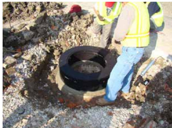
10. Place the Angle Ring onto the Finish Ring with the adhesive facing down, making sure to align with the previously applied paint mark.
