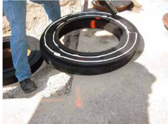
8. Apply M-1 as before to each groove on the underside of the Finish Ring and position with the grooves down onto the Grade Ring.
