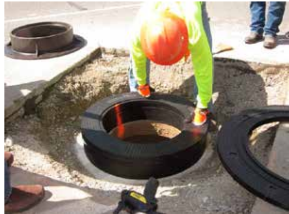
10. Place the Angle Ring onto the Finish Ring with the adhesive facing down, making sure to align with any previously applied marks.
