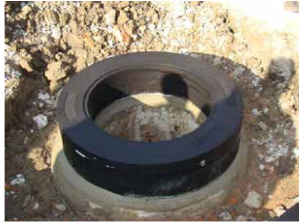
8. Apply M-1 as before to each of the tongues and position the Finish Ring with the grooves down onto the Grade Ring.
