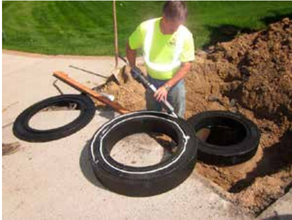
7. Apply a ¼" to ½" bead of M-1 adhesive to the groove and to the outer glue trench of the next Grade Ring or proceed to step 8 for Finish Ring
