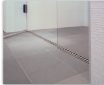
ProLine Drain at the Door Installation
