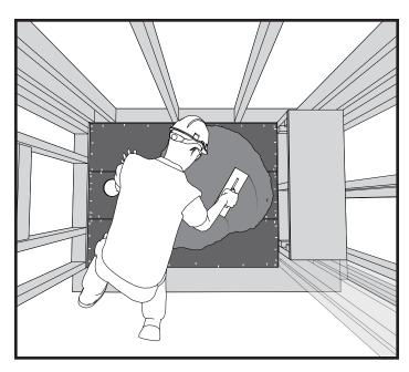
6. Spread your mortar base (should be a milk shake consistency), evenly across the subfloor at the thickness calculated in Step 5.
