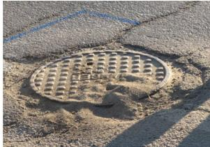
Aging sanitary collection systems are developing leaks. As a result, excess water is getting into the system. The added flow not only reduces sewage carrying capacity, but
