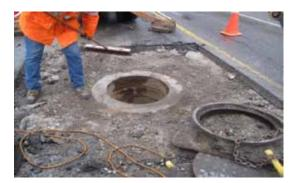
4. Drill through frame, ajustment risers, grade rings – then into structure Tap anchor bolts carefully into foundation structure (leave 2.5-4" of bolt exposed for frame and grade ring).
