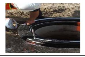
3. Drystack frame, adjustment risers, and grade rings ¼" below final street grade and mark their orientation (top of install needs to be even with eventual slope of the road).
