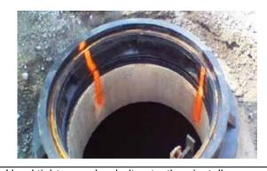
6. Hand tighten anchor bolt nuts, then install cover assembly using a torque wrench set to <u>35 ft/lbs.</u> Once cover is secured with cams engaged under frame, tighten anchor bolt nuts completely.
