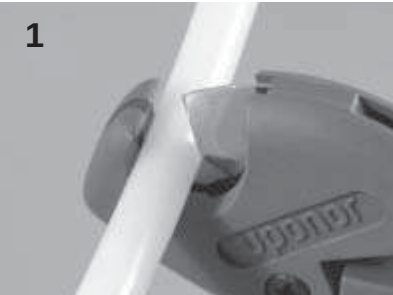
Square-cut the tubing
