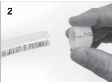
Slide ProPEX ring onto tubing
