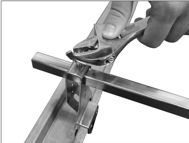
**NOTE:** For adjustment purposes, the wing screw on top of the Style AB2 end bracket assembly can be loosened to allow the end bracket to slide on the square bar. Tighten the wing screw on top of the end bracket assembly to a torque of 36 inch-lbs/4 N•m (approximately ½ to ¾ of a turn past hand-tight) to secure the end bracket to the square bar.
