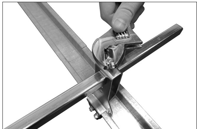
4. Verify that the wing screw on top of the end bracket assembly is tightened to a torque of 36 inch-lbs/4 N•m (approximately ½ to ¾ of a turn past hand-tight).
