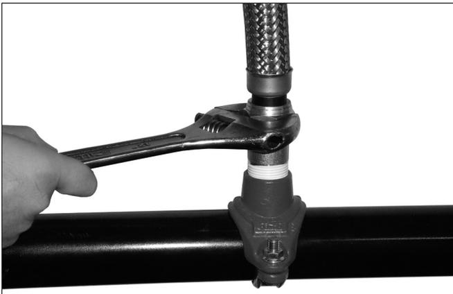
2. Confirm that the seal inside the nut of the flexible hose is in place and is free from damage prior to installation. Connect the nut to the adapter nipple, as shown above.
