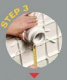
Measure distance from floor to stop inside of shower drain. Cut pipe to measured height.
