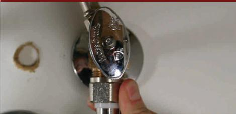
**Figure 7: Install Flex Line to Flange**
