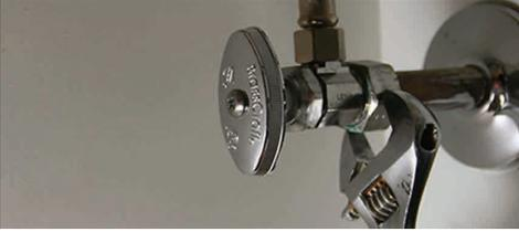
**Figure 4: Install T's and Re-attach Angle Stops**
