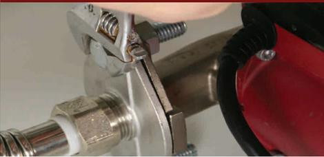
**Figure 6: Install Flex Line to T**
