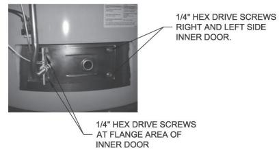
Step 8. Fully inspect inner door gaskets for the following:
