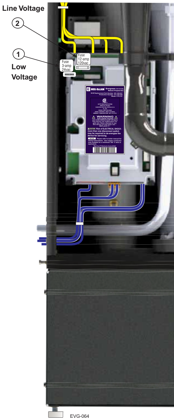
Figure 96 Control fuses
