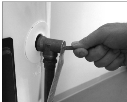
Figure 38 - T&P Relief Valve
