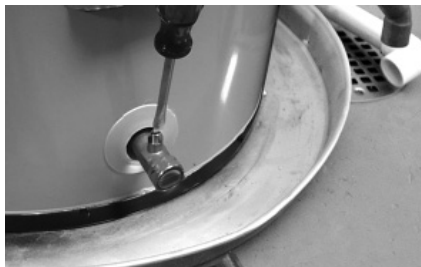
Figure 10 - Draining the old water heater.
