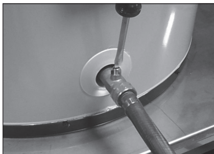
Draining the old water heater.
