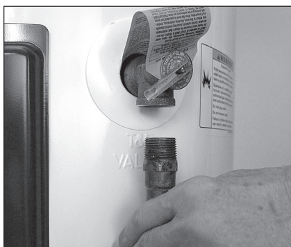
Removing the T&P Relief Valve discharge pipe.
