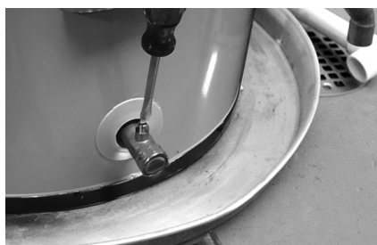
Figure 20 - Draining the old water heater.
