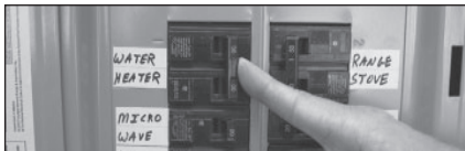
Figure 24 - Circuit Breaker
