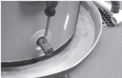
Figure 10 - Draining the old water heater.
