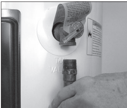
Figure 11 - Removing the T&P Relief Valve discharge pipe.
