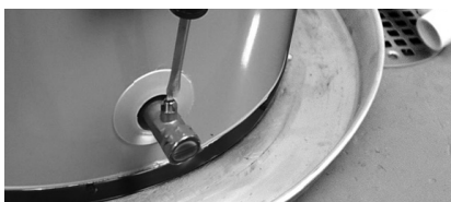
Figure 42 - Draining the water heater.
