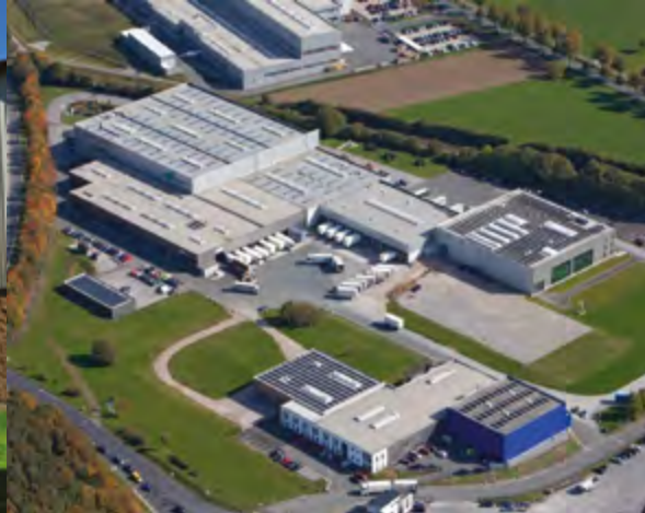
Centrotherm Systemtechnik GmbH Brilon, Germany
