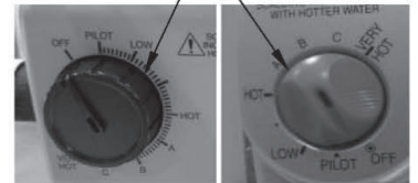
Gas controls shown in the "OFF" position
