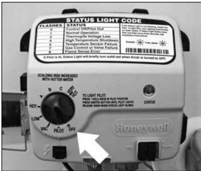
Figure 40 - Turn gas control/temperature knob OFF.
