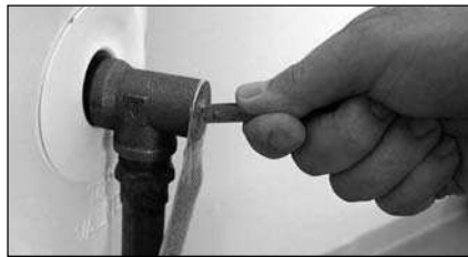
Figure 45 - T&P Relief Valve.
