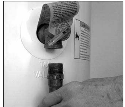
Figure 21 - Removing the T&P Relief Valve discharge pipe.
