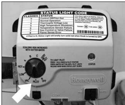
Figure 48 - Gas control/valve.
