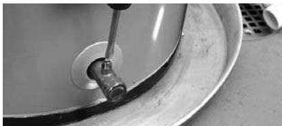
Figure 42 - Draining the water heater.
