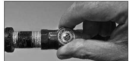
Figure 58 - Gas valve in "on" position.
