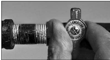
Figure 50 - Gas valve in "off" position.
