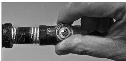
Figure 32 - Gas valve in "on" position
