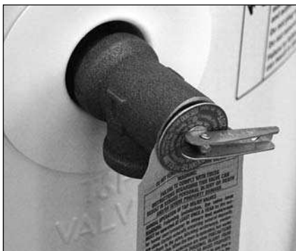
Figure 25 - Temperature and Pressure Relief Valve
