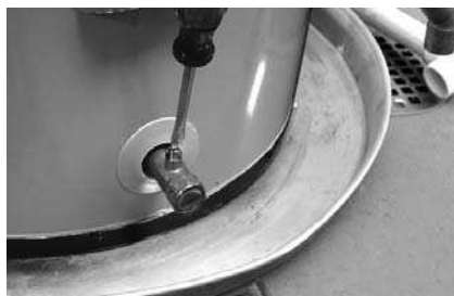
Figure 20 - Draining the old water heater.
