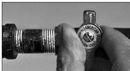
Figure 50 - Gas valve in “off” position.
