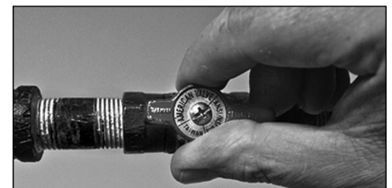
Figure 58 - Gas valve in “on” position.
