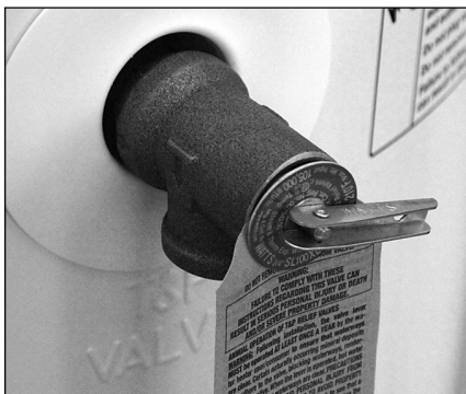
Figure 25 - Temperature and Pressure Relief Valve
