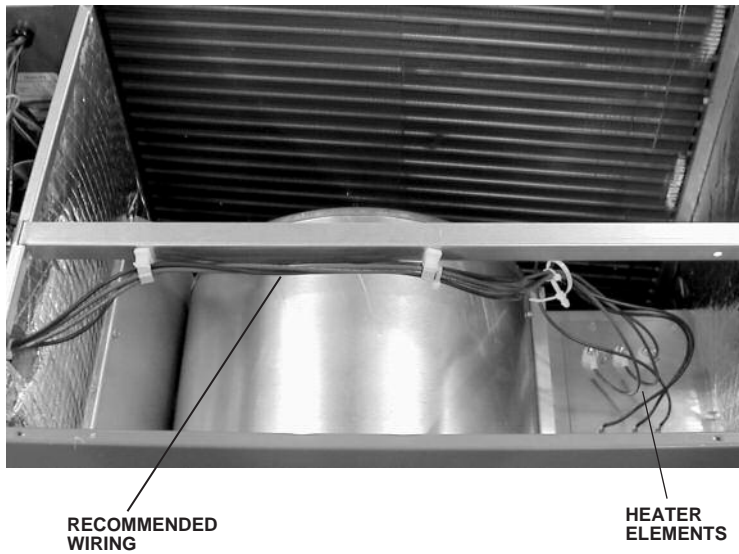
FIGURE 5 HEATER KIT INSTALLATION
