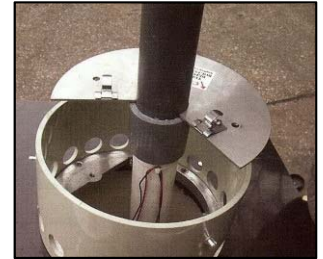
Pull up inner piping
