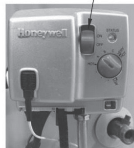
GAS CONTROL SHOWN IN THE "OFF" POSITION
