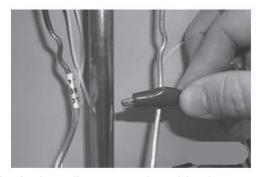
Step 4a. For White Rodgers Mechanical: to replace the igniter, disconnect the white (orange) wire from the igniter. Use a flat-head screwdriver under the igniter and gently pry bracket from the front of the gas calce and unhook the bracket from rear of the gas valve.
