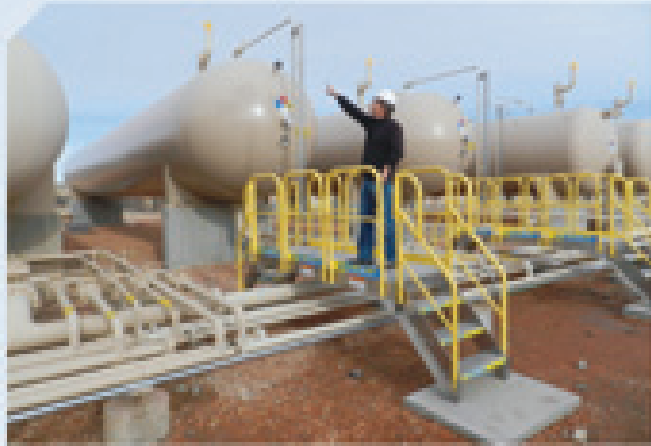
30" vertical clearance, 9' span over pipes.
